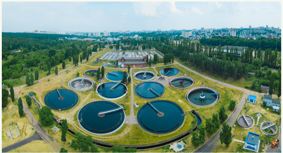
Photo 2: View of a wastewater treatment plant in 2022
